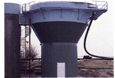
SLUDGE THICKENING AND RECIRCULATION IN AN ANAEROBIC BIOGAS PROCESS.
