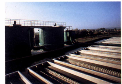
RESTORATION OF A HEAVILY CONTAMINATED INLAND LAKE.
