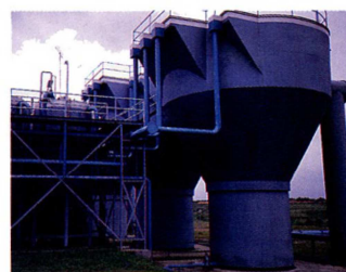
THE JOHNSON LAMELLA SEPARATOR.
