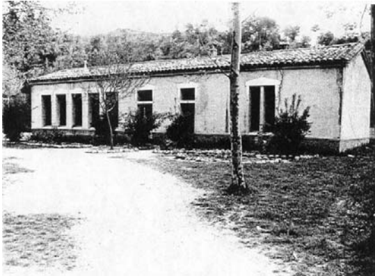
Façana principal any 1955
