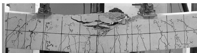
Figure B-102. Crushing of concrete for C2-212-D1-B.
