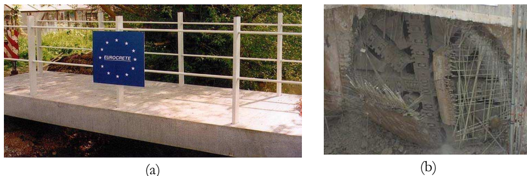
Figure 1-1. Applications of FRP to RC elements: (a) The first concrete footbridge in Europe with only FRP reinforcement (EUROCRETE project) (b) Soft eye FRP reinforcement (fib 2007).
