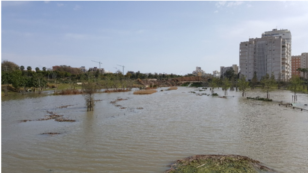
La Marjal Flood Park (Playa de San Juan, Alicante): (a) empty, (b) with 15,000 m3 of flood water produced by the event of 13 March 2017). Source: Aguas de Alicante (reproduced with permission)
