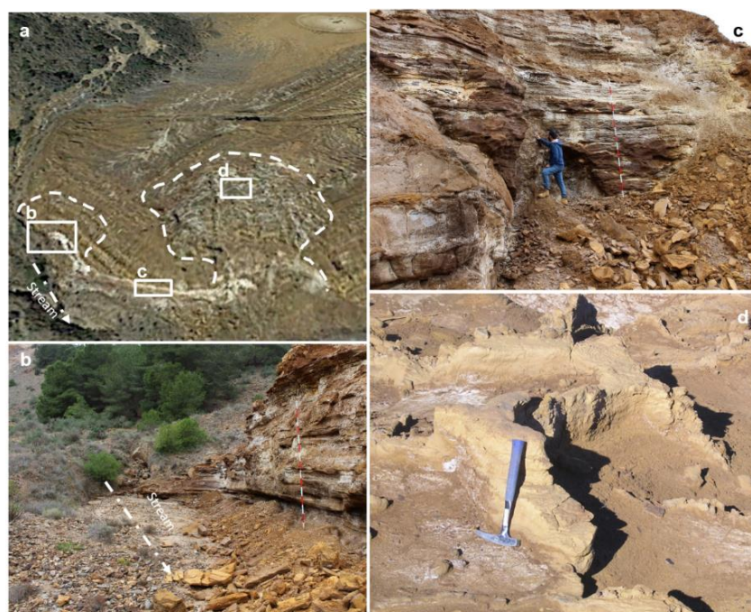
Figure 8. (a) Oblique view of landslide one (LL1) and two (LL2); the discontinuous arrow indicates the direction of the stream runoff; source Spanish National Geographic Institute-IGN and Google Earth© landslide one. Detailed views landslide one (LL1) (b) and landslide 2 (LL2) (c). (d) Sand dikes exposed on the surface of landslide two (LL2).
