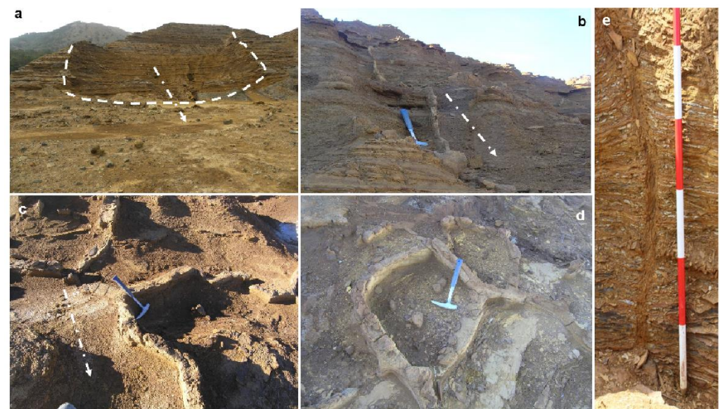
Figure 11. (a) View of the breach in the wall of the impoundment in landslide four (LL4). (b) Close-up view of a sand dike cross cutting the subhorizontal tailings bedding. Plan view of the polygonal arrangement of sand dikes on the LL4 surface (c) and lagoon four (Lg4) (d). (e) View of a sand dike exposed on the breach plane of landslide five (LL5). The discontinuous arrow indicates the direction of the runoff.
