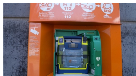
Figure 8 Fixed AED from the “GTC” project (51)
