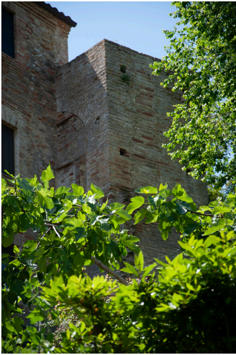
Fig. 7. The first tower of the western walls.
