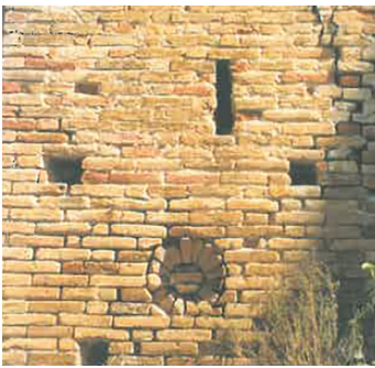
Fig. 8. Radiating loophole in the first tower of the western walls.
