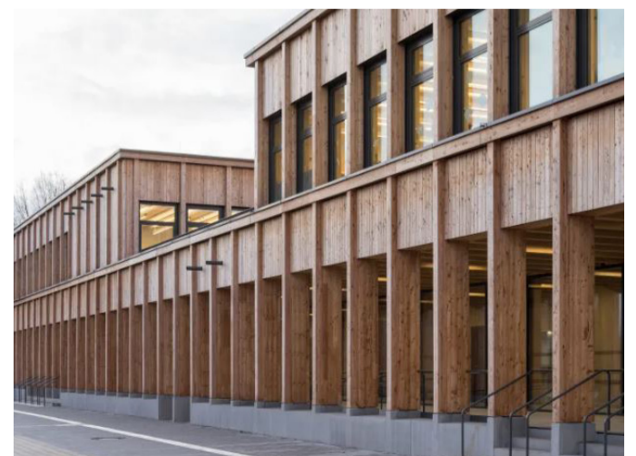
INTEGRATED COMPREHENSIVE SCHOOL IN RINTELN
