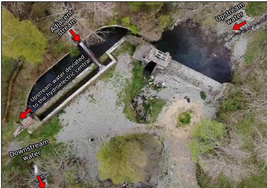
Figure 2. Hydroelectric dam of the Catllar stream. Upstream water is deviated to the hydroelectric power station. Downstream water comes from an adjacent stream that falls into an underground passage.
