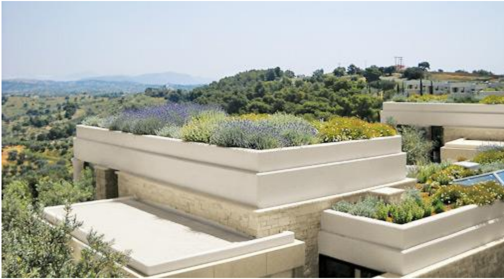
Fig. 6: Coberta semi-extensiva (Zinco, 2018)
