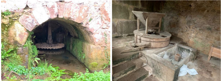
Figure A2. Water mill completely rebuilt in the Colomer farm
