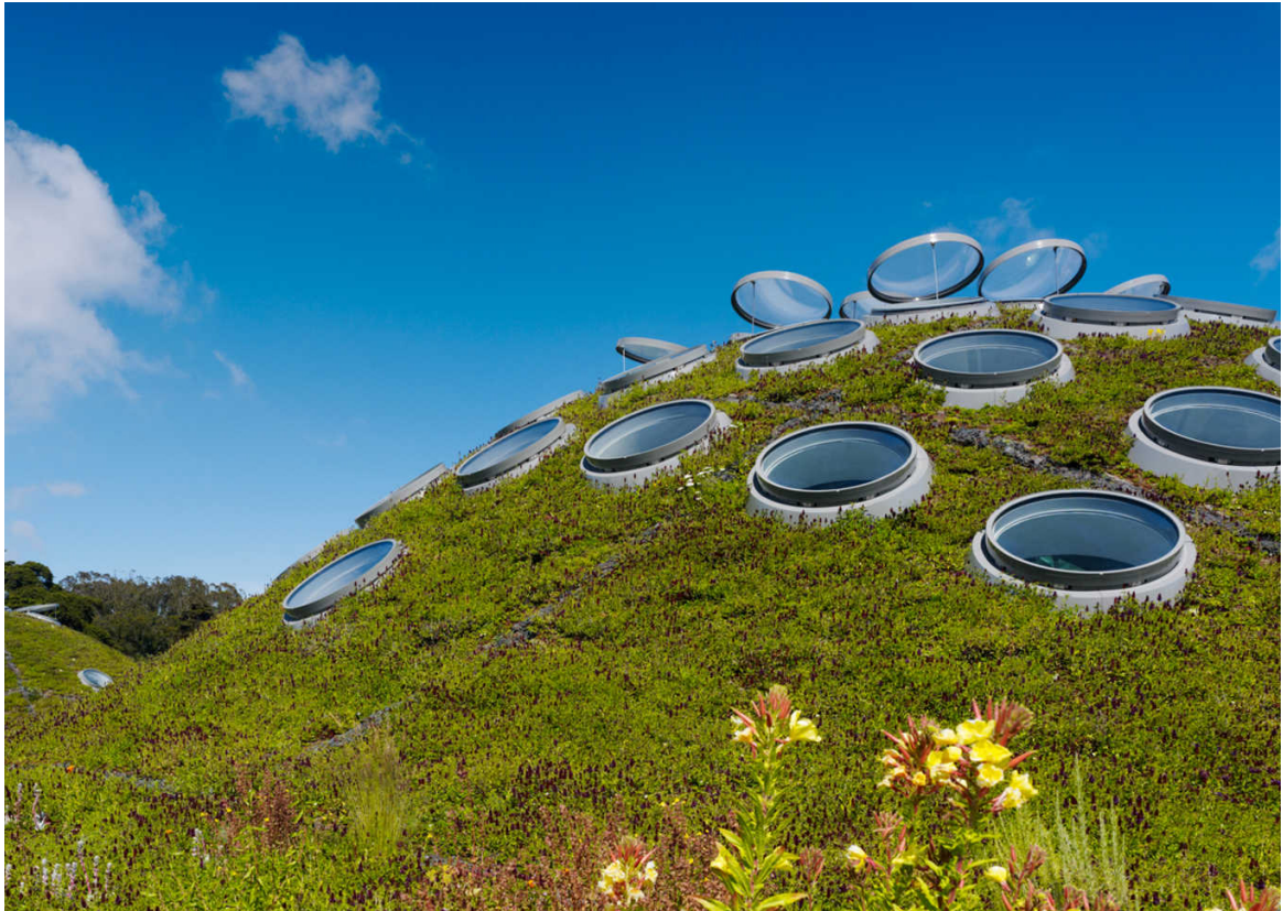
California Academy of Sciences. Imatge extreta de https://www.calacademy.org/about-us/sustainability-in-action/green-building-operations
