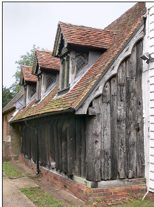
Figure 2. Garbutt, S. (2009). Stave church at Greenstead in Essex, England. [North wall and west wall originally from the 9th century]. [Digital Image] Retrieved from: https://en.wikipedia.org/wiki/Greensted_Church#/media/File:Greensted_Church_North_Side.jpg
