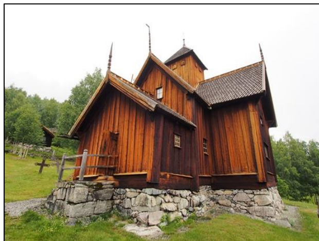
Figure 4. Uvdal stavkirke [An example of an early stave church. We can observe the stone foundation that lies under the church.] (2018) Retrieved from: Fortidsminneforeningen: https://fortidsminneforeningen.no/avdelinger/nyheter-buskerud/uvdal-stavkirkes-850-arsjubileum
