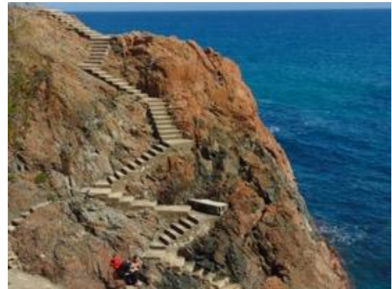
Fig. 32 – Stairs leading to the beach in the coastal path of S'Agaró
