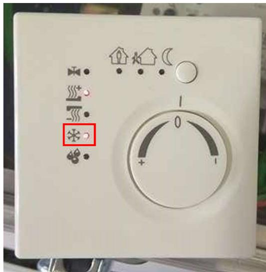
Figure 114 - KNX Room temperature controller (Frost protection mode)
