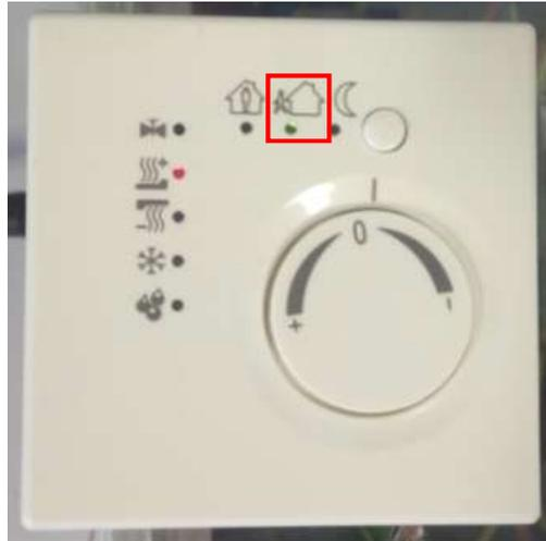
Figure 115 - KNX Room temperature controller (Standby mode)
