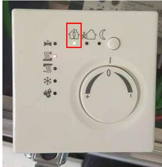
Figure 113 - KNX Room temperature controller (Comfort mode)
