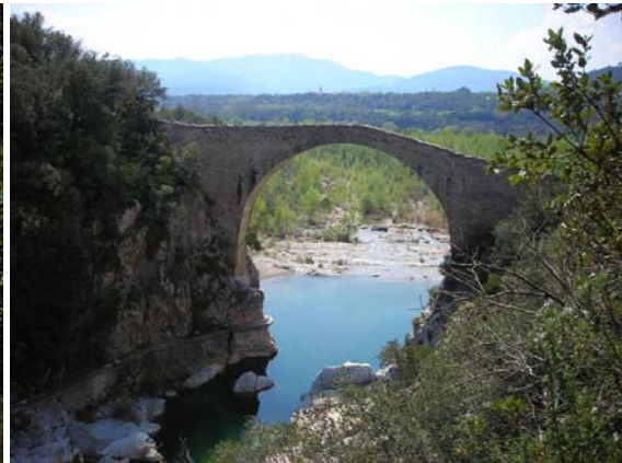
Picture 12: The Sadernes bridge.
