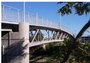
Figure 1.1 Sherbrooke bridge, Canada 1997
