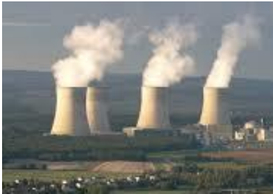
Figure 1.5 Cooling towers of Cattenom, France 1999
