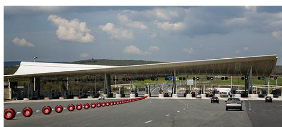
Figure 1.4 Tollgate canopy Viaduct-de-Millau, France 2004
