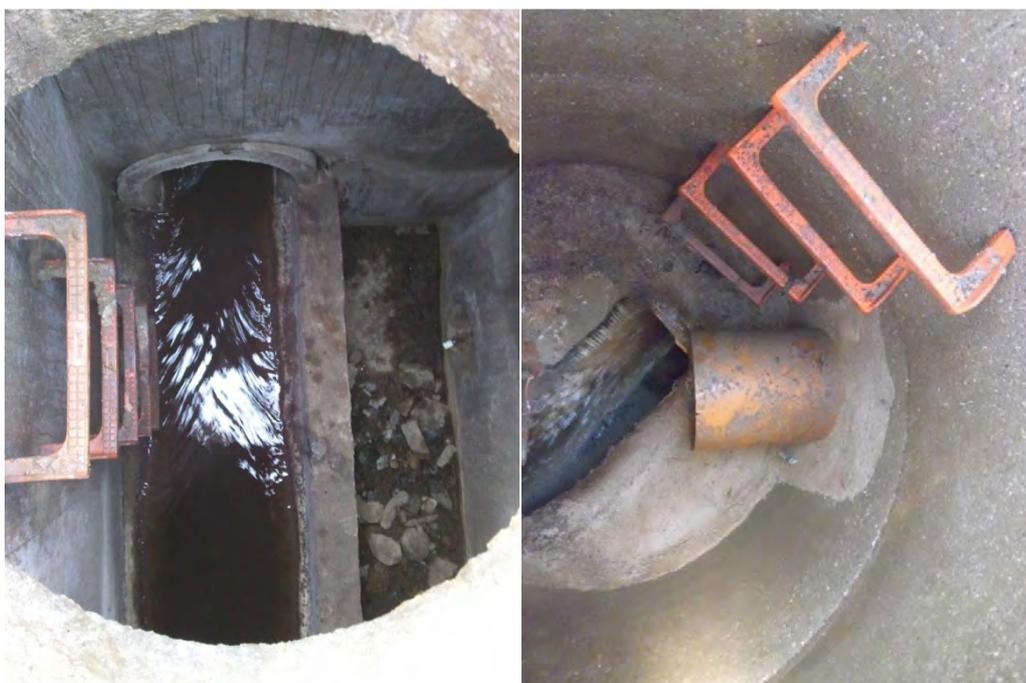
**Figure 3-3.** Examples of side weir (left) and transverse weir (right) from the CSS of La Garriga.
