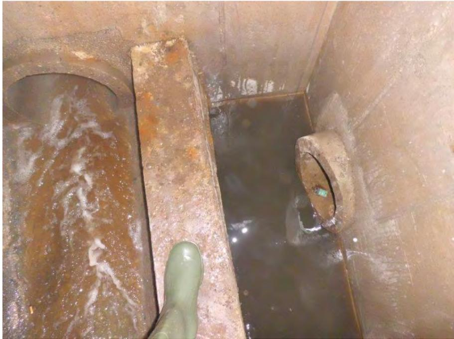
**Figure AII-3.** Detail of the CSO Structure 13. As in the case of Structure 11, part of the CSO remains in the channel of the side weir during dry weather conditions.
