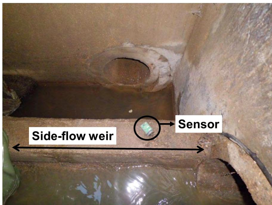
**Figure AI-3.** Detail of the sensor installation on the crest of a side weir.
