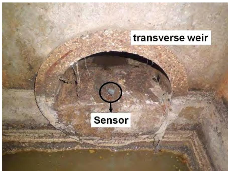
**Figure AI-2.** Detail of the sensor installation at the bottom center of a transverse weir.
