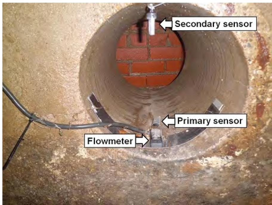
**Figure AI-4.** Installation setup for the verification of the method consisting on a flowmeter, a primary and a secondary temperature sensors.
