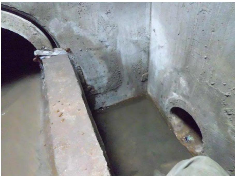
**Figure AII-2.** Detail of the CSO Structure 11. It can be appreciated stagnant water in the channel of the side weir during dry weather conditions.
