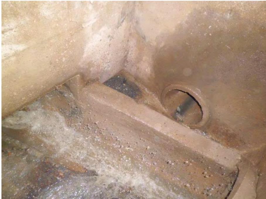
**Figure AII-1.** Detail of the CSO Structure 9. It can be appreciated the water turbulence created by a drop structure.
