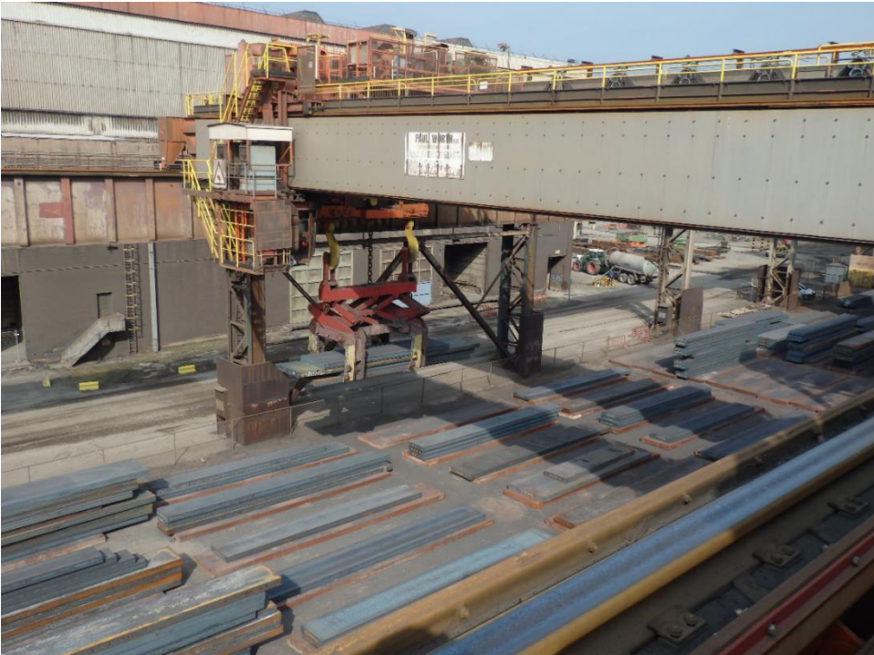
Figure 4.1 One of the overhead cranes analysed in the project.
