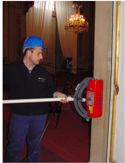
Fig. 8. Georadar survey performed inside the “Sala delle Nicchie” using the HIRESS system.
