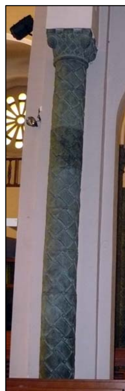
FIG 2: Pilar de pedra artificial
