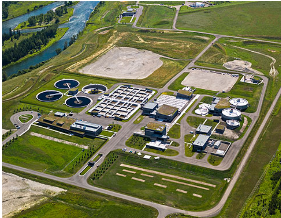
Figure 2. Aerial picture of a Wastewater treatment plant.
