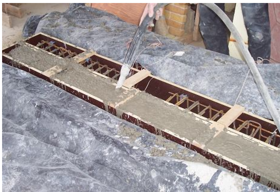
Figura 14: Formigonat C2, in situ
