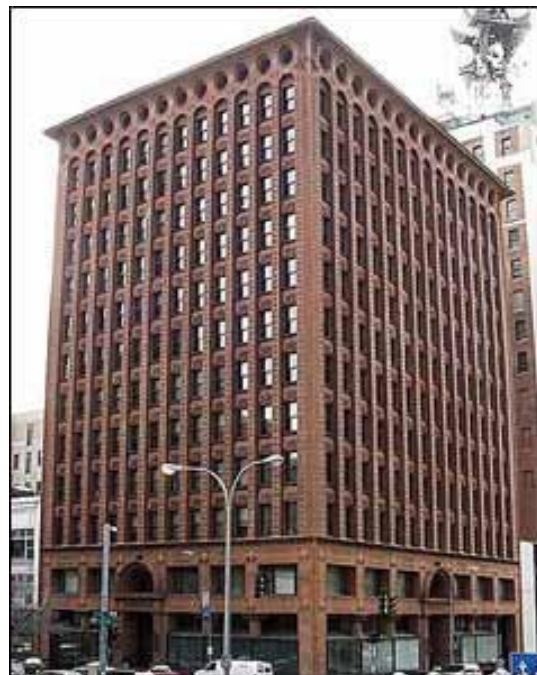
Guaranty Building, 1895. Adler & Sullivan
