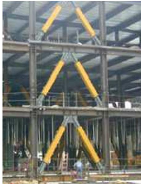
Figure 2: Section of buckling restrained brace (Open Steel Joists)
