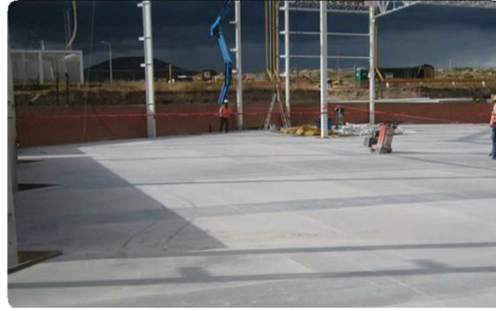
Industrial floor - OC Puma plant, Mexico. 10 kg/m 3 Anti-CRAK® HP 67/36 + 0.6 kg/m 3 Anti-CRAK® HD12, C 25/30
