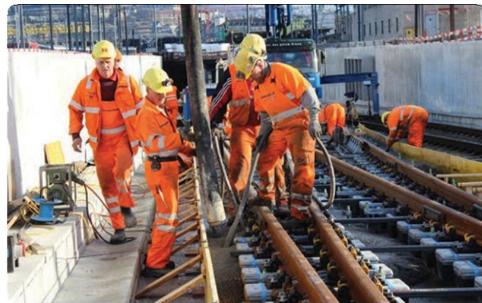
Railway base - Zurich Diameter Line, Switzerland. 8kg/m 3 Anti-CRAK® HP67/36, C25/30
