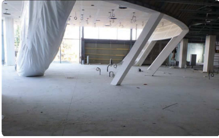
Commercial floor - Audi dealership, France. 5 kg/m 3 Anti-CRAK® HP 67/36 + 0.6 kg/m 3 Anti-CRAK® HD12, C 20/25.
