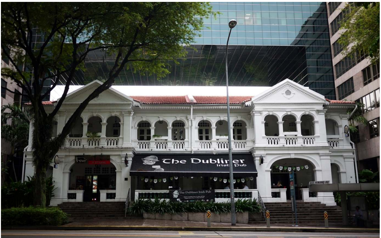
Illustration 2-37 Historical building framed by contemporary structures, Singapore (Author, 2011).
