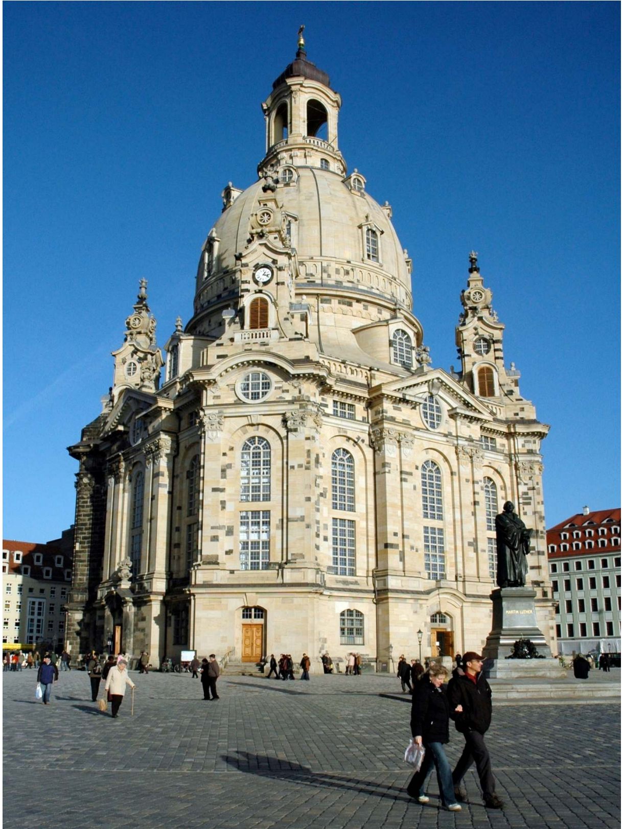
Illustration 2-16 Church of Our Lady (Frauenkirche) Dresden, Germany: The remaining parts of the original are still visible as dark spots within the rebuilt structure (Author, 2006).
