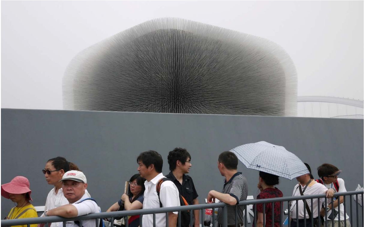
Illustration 2-51 UK pavilion at Expo 2010 in Shanghai, China: The structure costing £15 million to be built was dismantled after the event (Moore, 2010) (Author, 2010).
