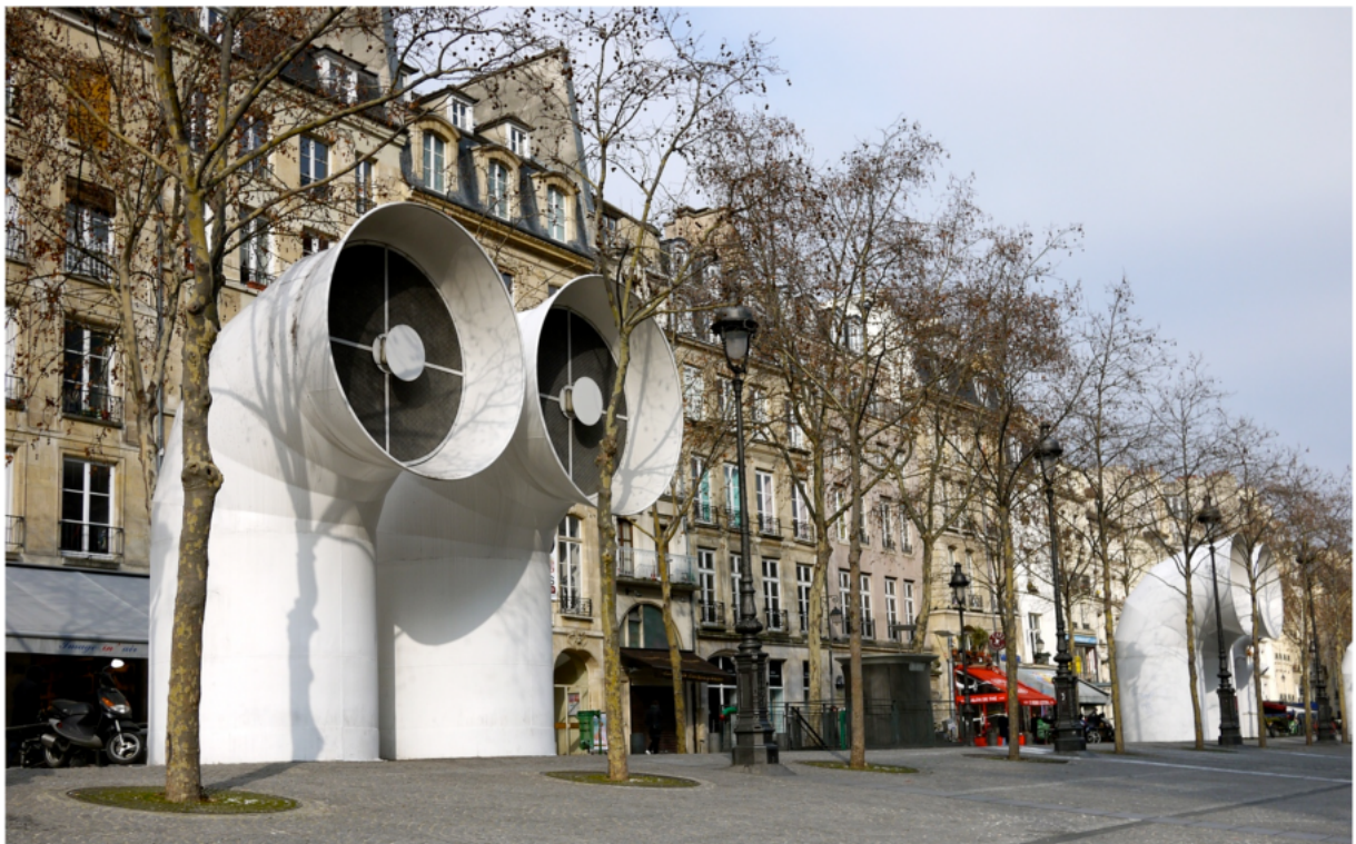
Illustration 1-3 Striking technical installations of the Pompidou Centre contrasting the “classical” built environment of Beaubourg, Paris, France (Author, 2009).
