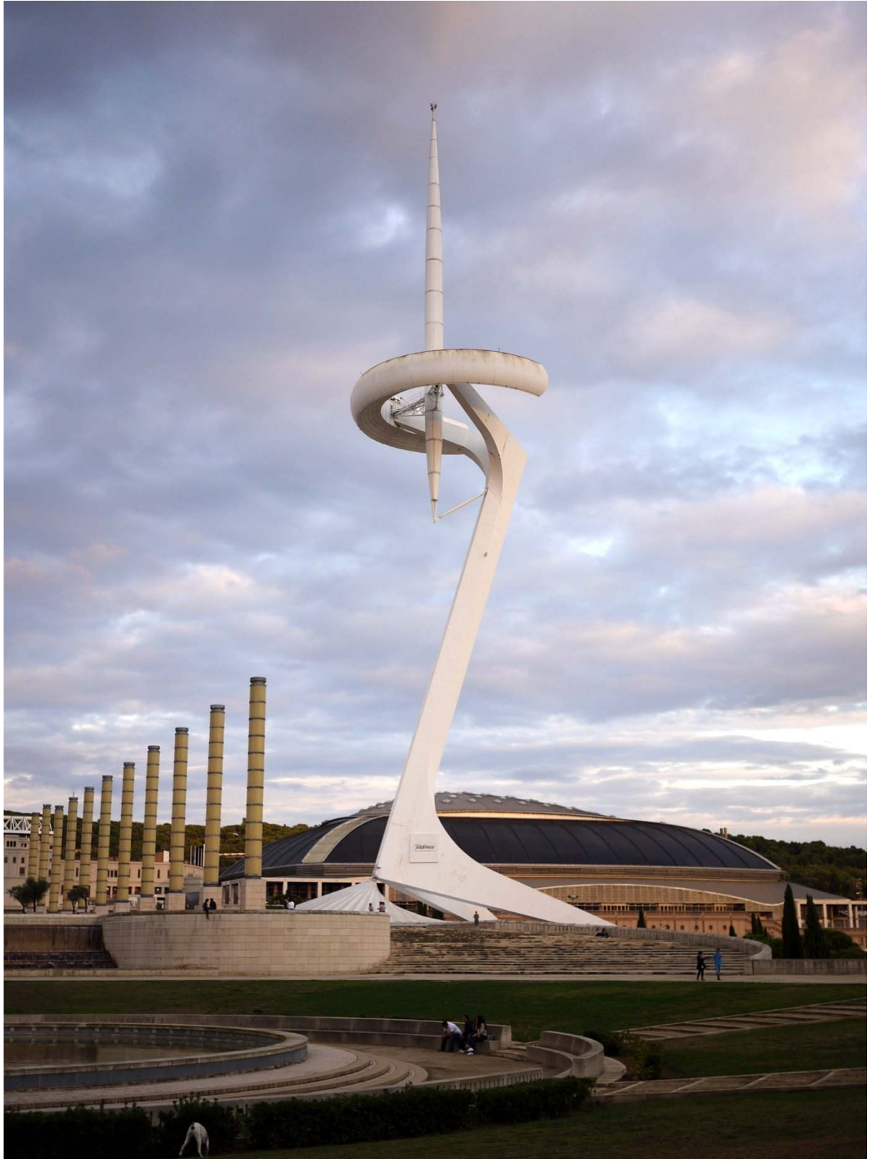
Illustration 2-32 La Torre Calatrava, Barcelona, Spain: Art or Architecture? (Author, 2011).
