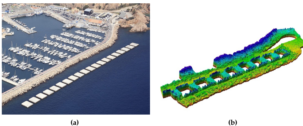
Figure 3. (a) breakwater structure in the harbor of Sant Feliu de Guíxols in Catalonia, Spain. The structure is composed of a series of blocks, each of which is 14.5 m long and 12 m wide; (b) Octomap created from real-world data obtained with a multibeam sonar.
